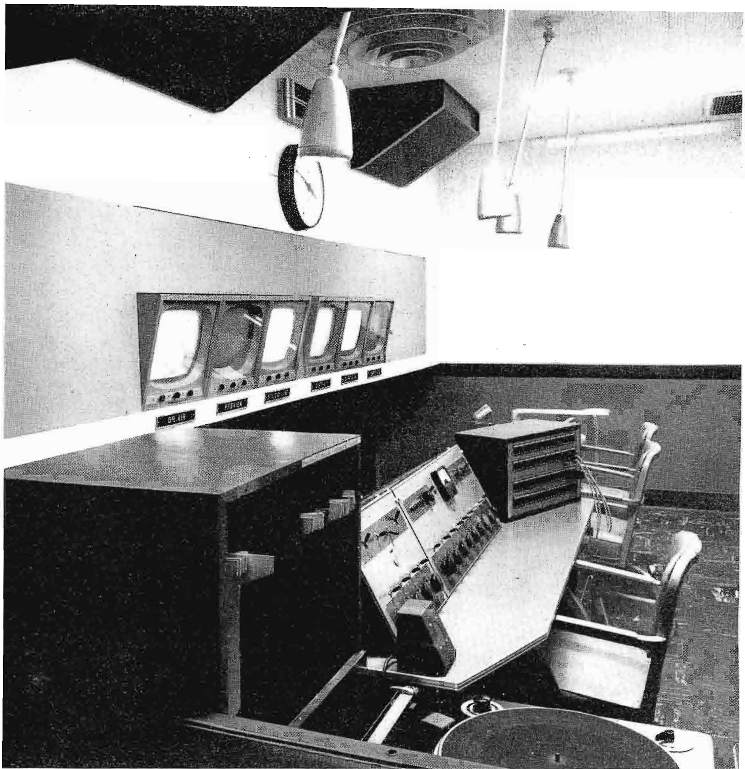
FIG. 24. View of a control booth from clients' booth. Audio position includes RCA BC-2B Audio Console and RCA BCM-11A Mixer Console, and two RCA BQ-70B Transcription Turntables.
