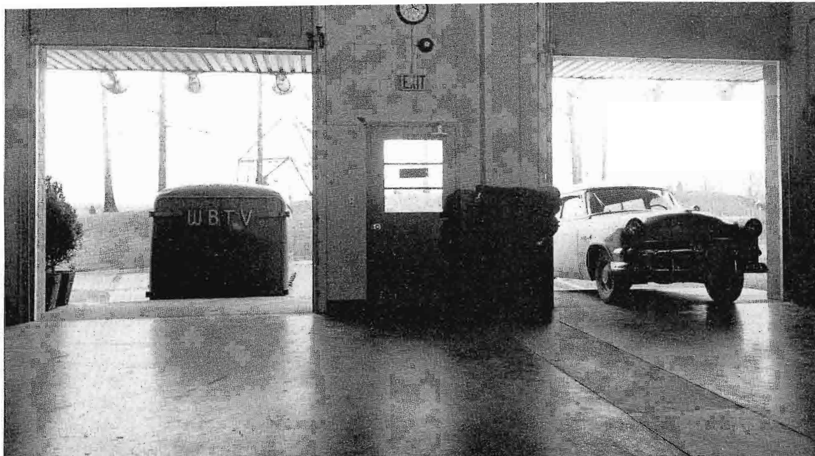
FIG. 13. One of the overhead doors from the prop area opens onto a loading dock which enables props to be rolled from a truck floor to the studio floor without lifting. The other door leads to a ramp which allows cars to be driven directly onto the floor of the studios.
