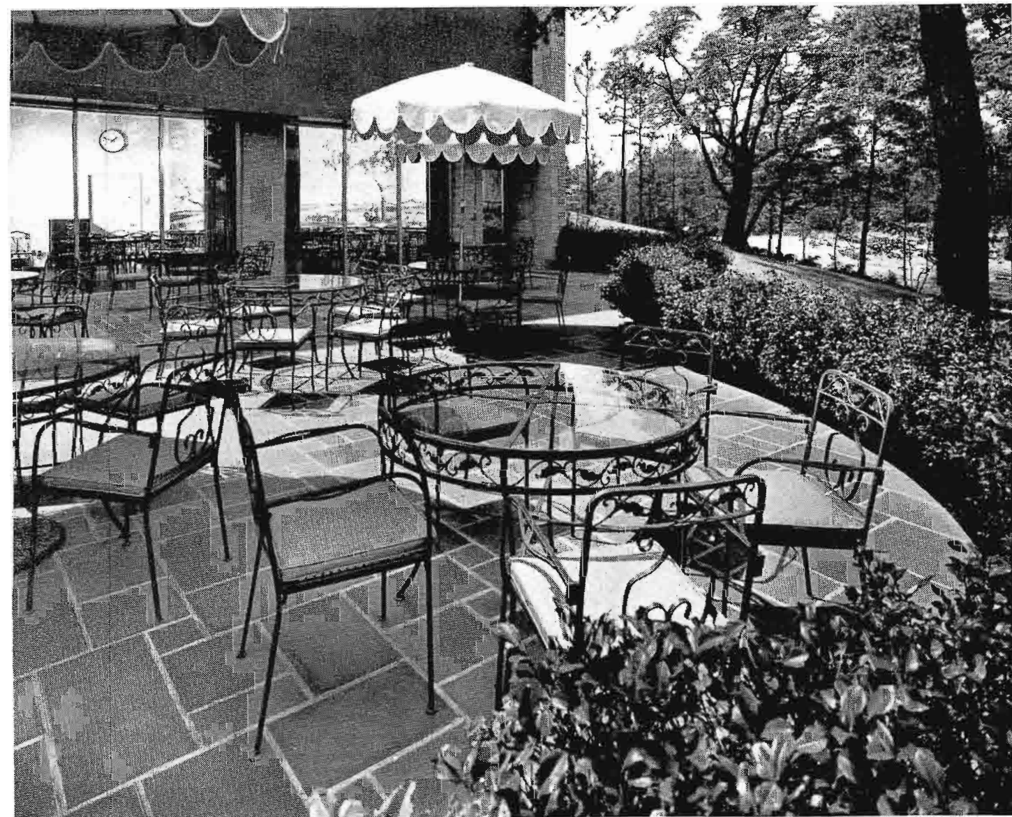
FIG. 50. In nice weather employees enjoy this beautiful dining terrace, which opens off the indoor cafeteria-dining area seen through the glass panels at rear.
