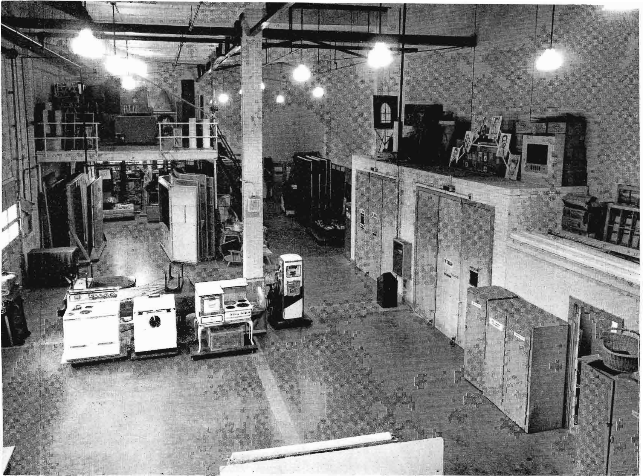
FIG. 10. This large (40-foot by 120-foot) prop construction and storage area is a feature of the WBT-WBTV Building. Large folding doors, at the right, open directly into the two tv studios. Overhead doors, at the left, open onto a loading dock and ramp. This area has the same ceiling height as the studios. Footings, which can be seen in the floor of this area, make it possible to enlarge either or both studios in 20-foot increments by moving non-load bearing studio wall to use part of present prop area.
