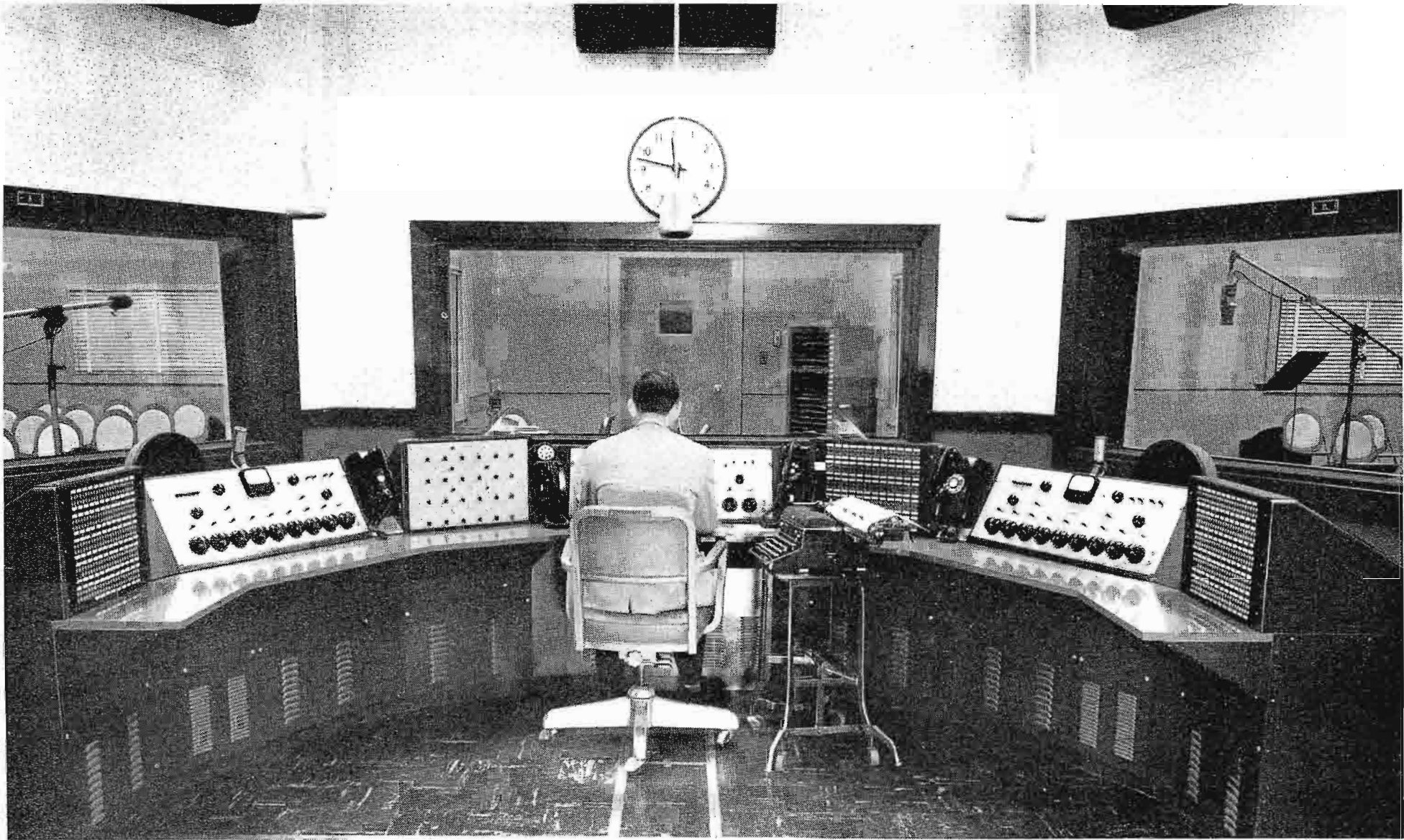
FIG. 45. Master control room of WBT looks into the three radio studios through conveniently placed windows. Master console includes a separate control panel for each studio plus terminal and switching facilities. Studio B (center) is a d.j. studio, equipped with four RCA Type 70-D Turntables and one announcer's control box.
