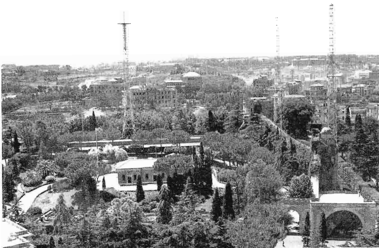
FIG. 24. Vatican transmitter building, showing partial view of antenna system. This building houses eight transmitters.
