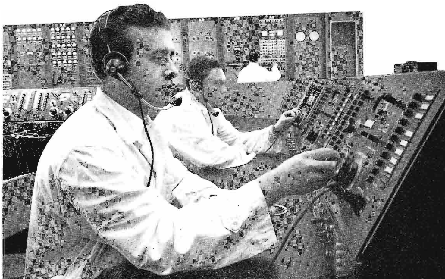
FIG. 21. Operators Vincent Minelli and Nicola Mancini at two of the master control positions.
